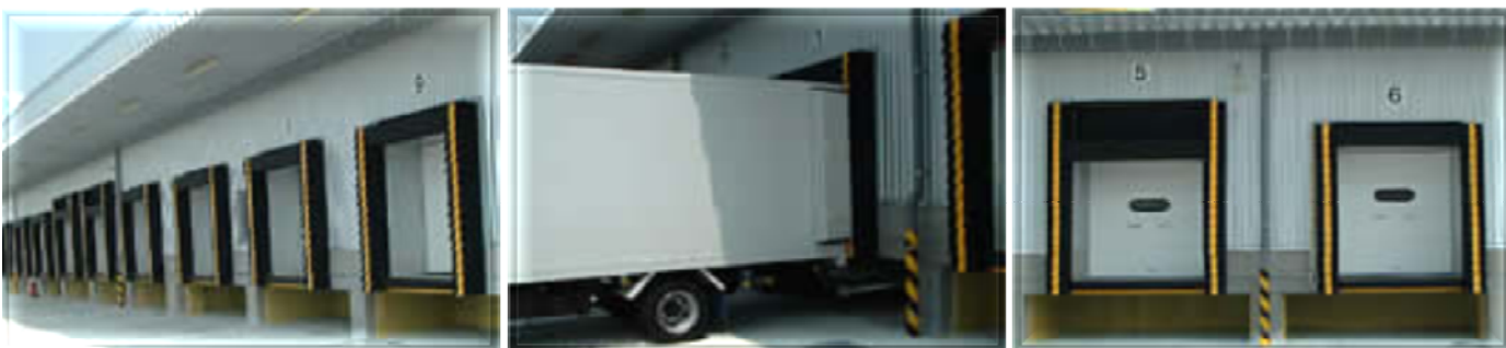
Examples of Construction of Armor Dock Shelter
